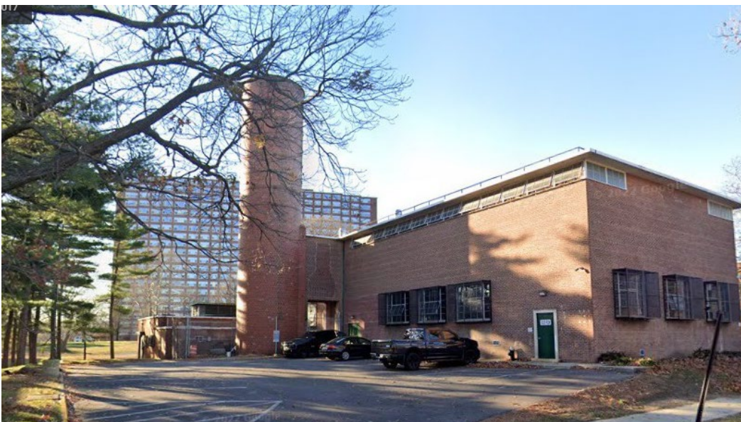
Figure 2. Boiler Facility at 67-19 192nd Street, Fresh Meadows
