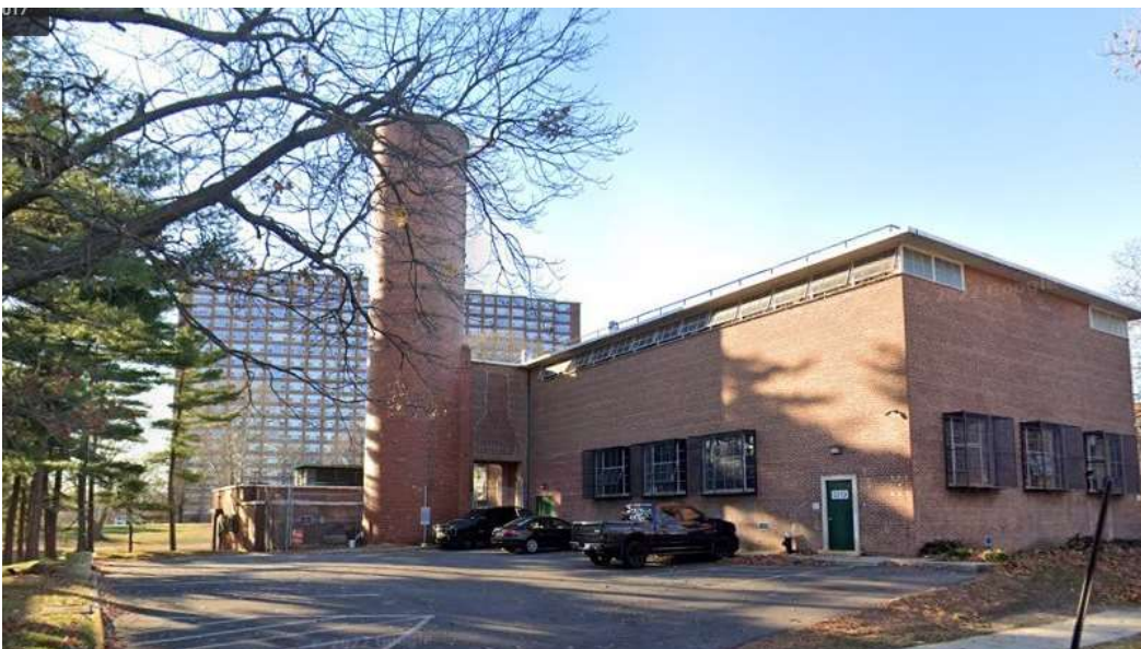
Figure 2. Boiler Facility at 67-19 192nd Street, Fresh Meadows
